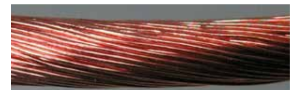
A close-up of the completely intact copper conductor. The inspection performed over the entire length shows that the conductor is still completely intact and does not have any individual wire breakages.
