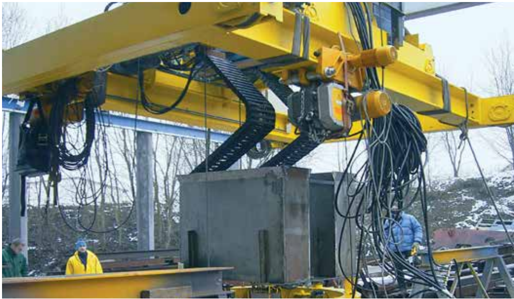
Decommissioning of a nuclear power station. Zig-zag application with igus® e-chains®
