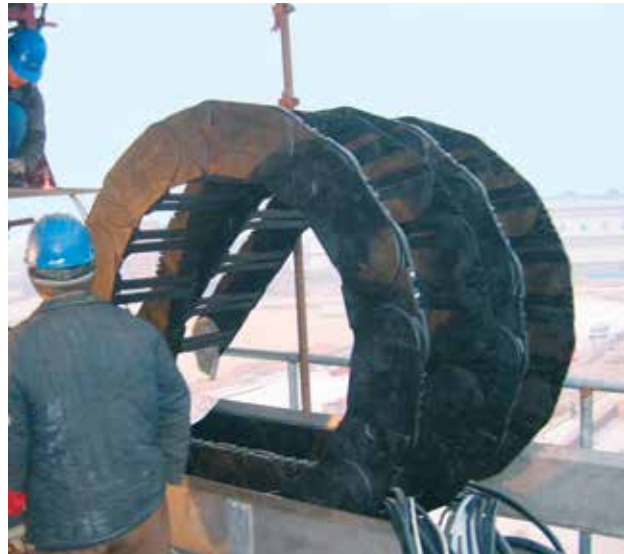
Assembling of an E4 e-chain® Series 800 in an igus® steel guide trough
