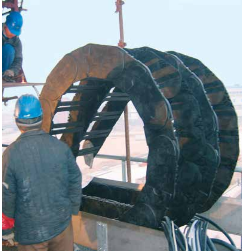
Assembly of an E4 e-chain® series 800 in a steel guide trough
