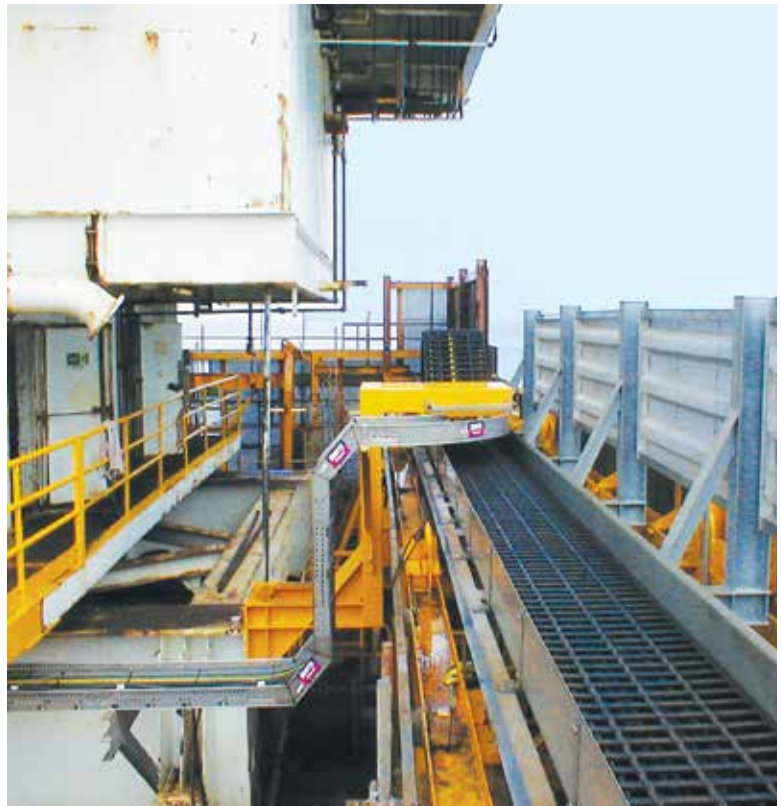
E4 e-chain® with several extension links for extreme fill weights, guided in igus® steel trough over long distances and in rough seas
