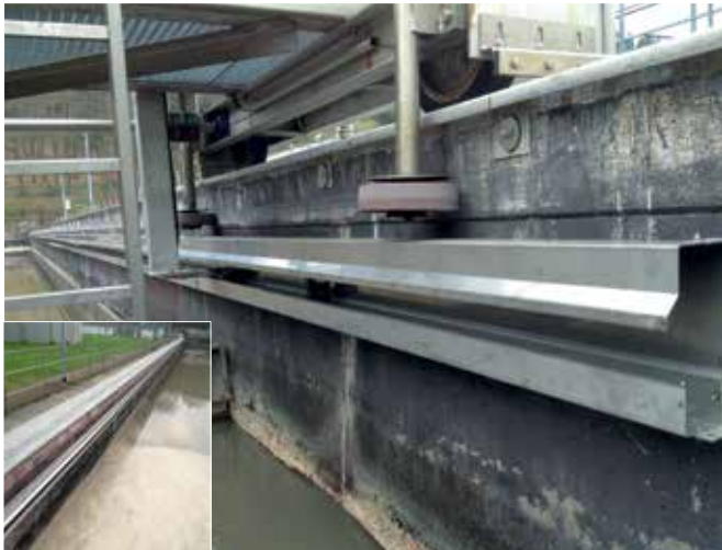
Longitudinal scraper, mounted in the basin, sewage treatment plant in Plauen, Germany - travel 174 ft (53m)
