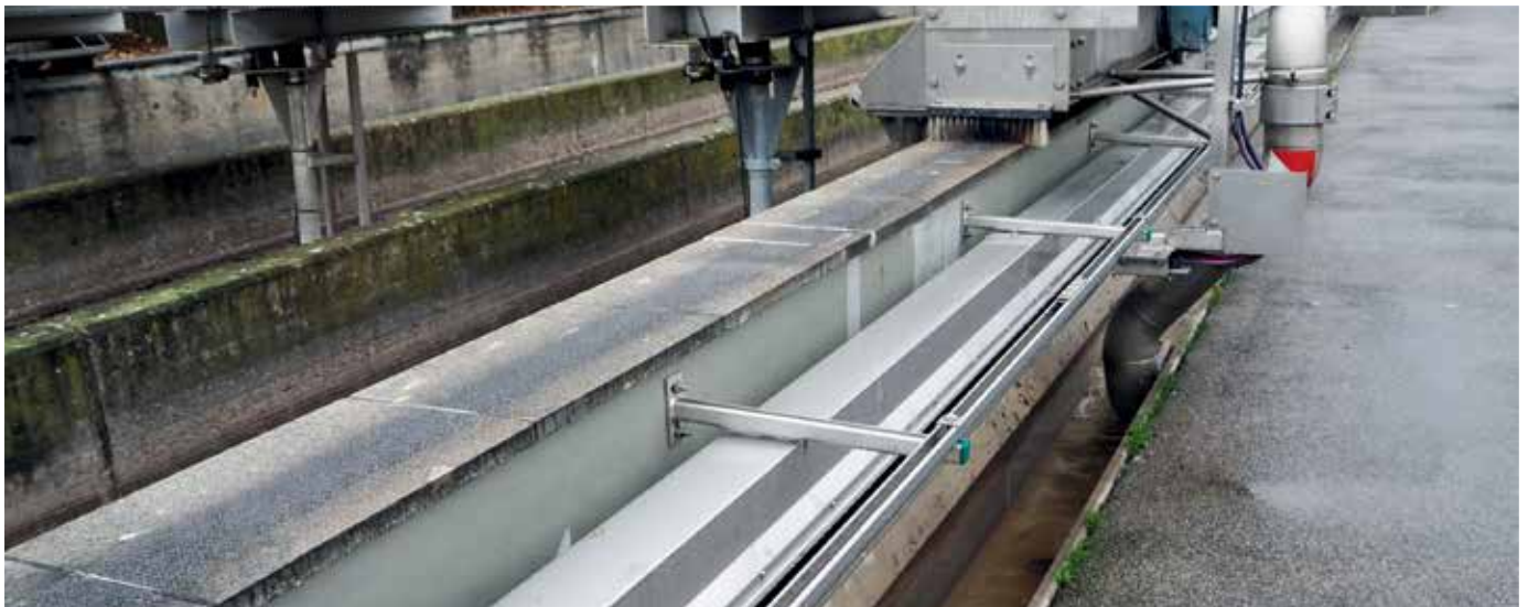
Sand traps, sewage plant in Bamberg (Germany) - travel 85.31ft (26m)
